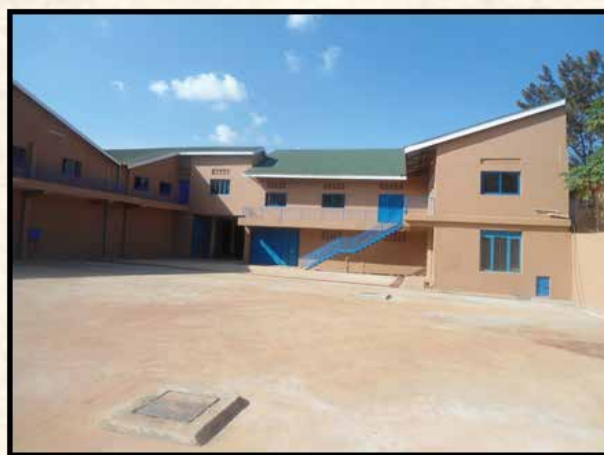
PROJECT TITLE: 5000sqm of Warehouse LOCATION: M275 Ntinda Industrial Area Kampala Uganda COMPLETED: April, 1999
